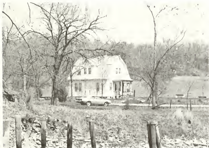
Former locktender's house directly north of Lock 11 and now a private residence. The house was moved from south of the lock to its present location in the 1960s.
